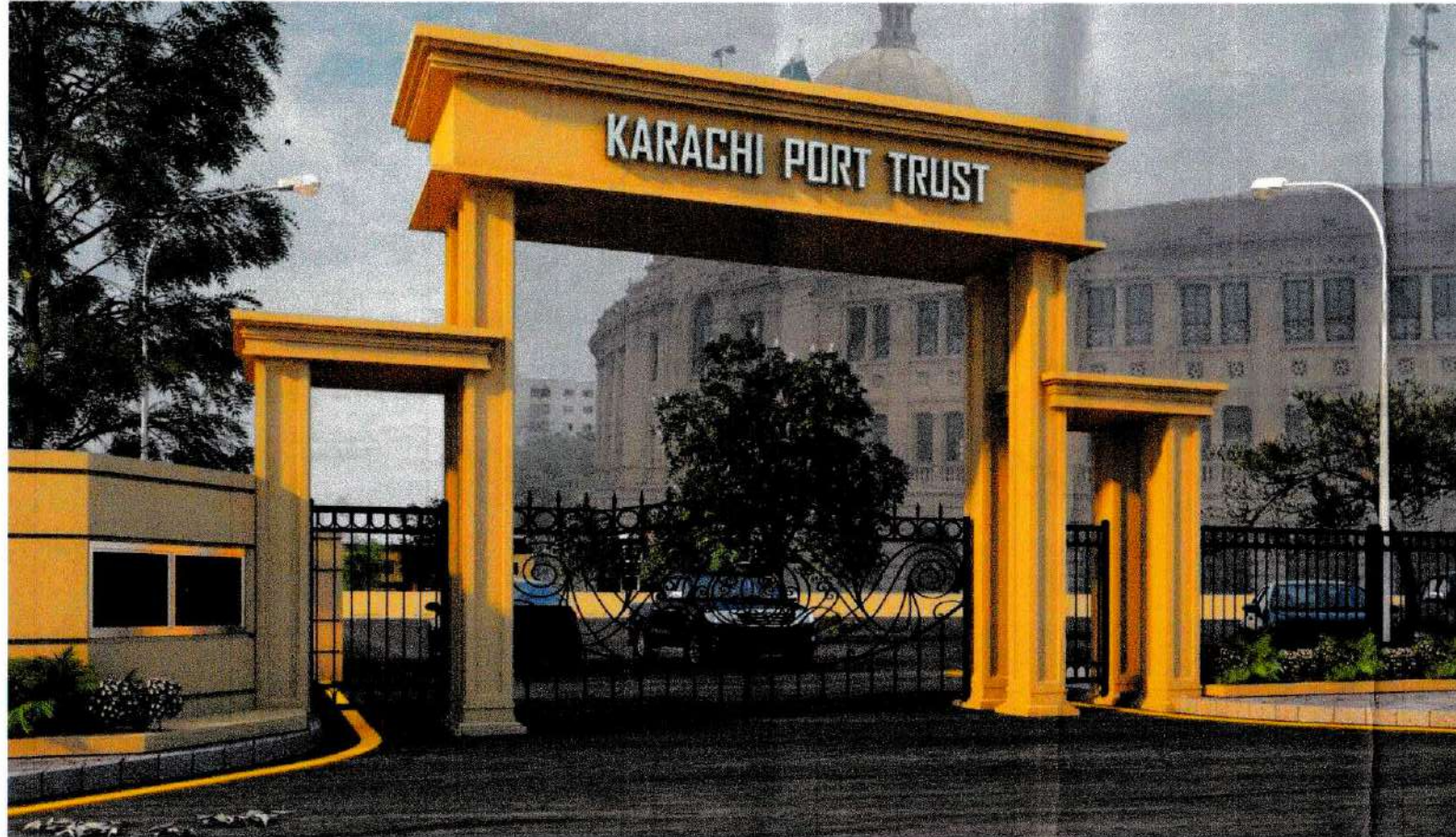
MAIN GATE 3D VIEW
